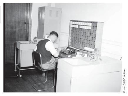
Don Beresford at keyboard control for tape punch. (L–R) Tape punch, cabinet with control circuitry, tape library, tape reader. 1958.
