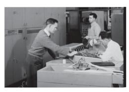
A new magnetic disc was installed replacing the magnetic drum used in Sydney. It arrived in Melbourne with the Mk1 without magnetic surface and several weeks were spent investigating a way of spraying a rotating disc with magnetic paint so that the surface was free from occlusions. The resultant magnetic disc gave excellent service. The new disc had a 1024 word capacity per side. The second side was not utilised until 1962 following extensive transistorised additions to the original circuitry.
